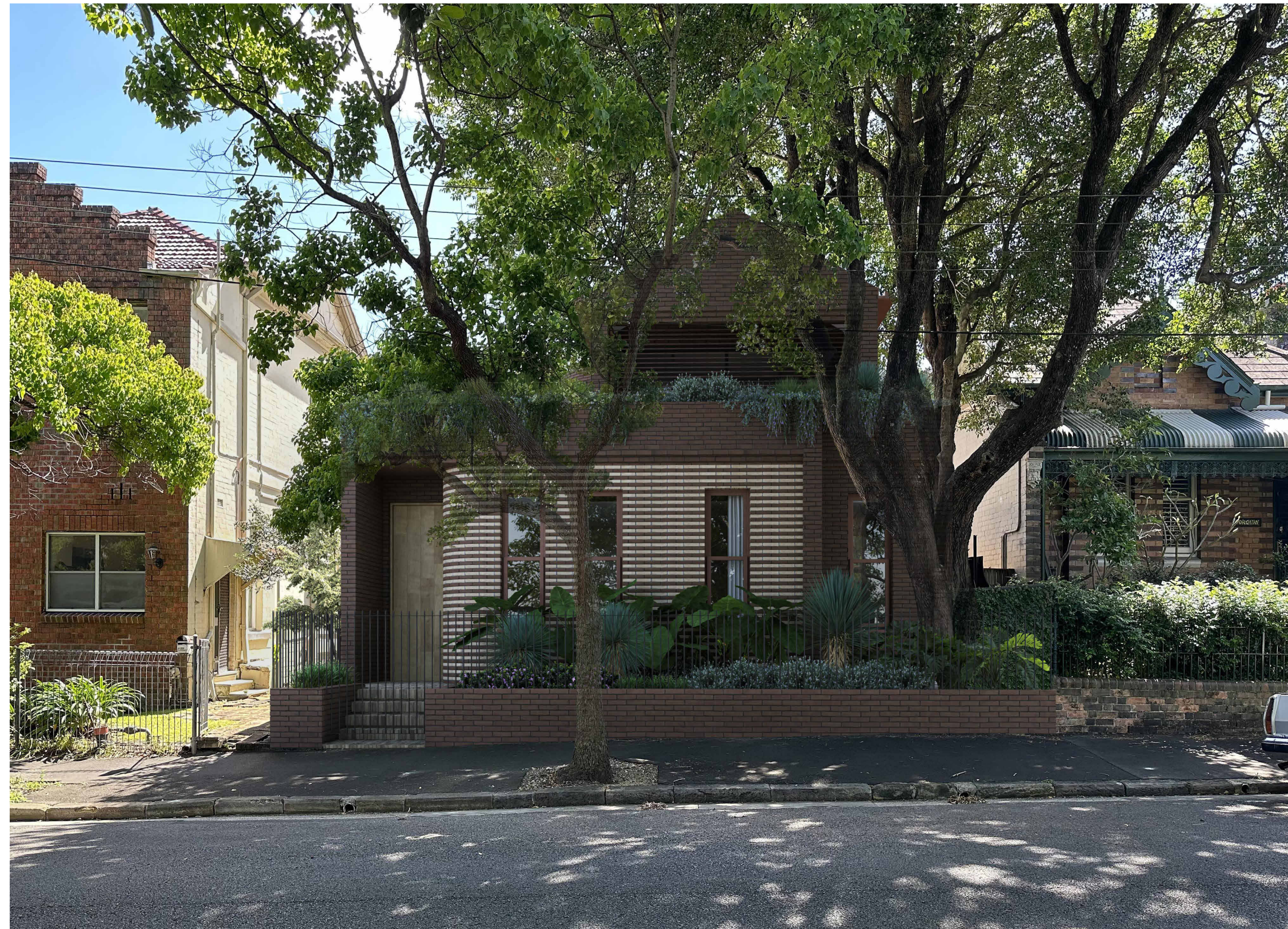
FRONT VIEW FROM ALLEN ST
